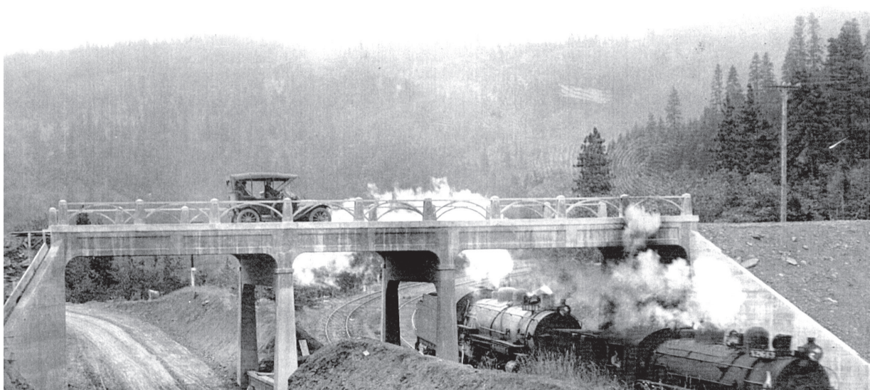
The Pacific Highway crossed both over and under the bridge and crossed the railroad tracks at the Steinman Overcrossing on the Oregon side of the border. This section of road is still drivable today.
