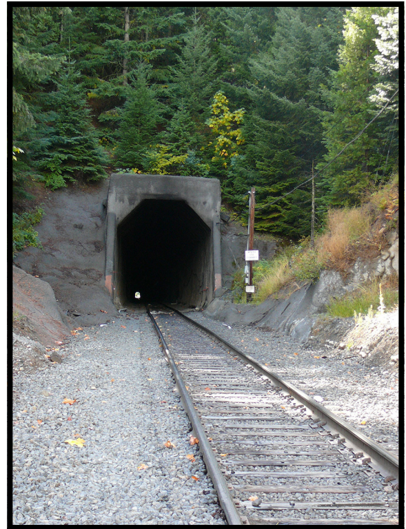
The railroad crossed the top of the Siskiyou in Tunnel 13, site of the country’s last train robbery.
