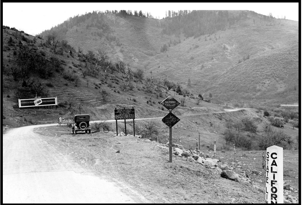
The thin layer of asphalt pavement on the Pacific Highway in Oregon ended right at the California border, as seen in this photo.
